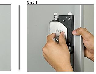
Open locker door, loosen and remove the nuts on the back of the hasp. Then remove the lock cover plate and the screws from the hasp.
