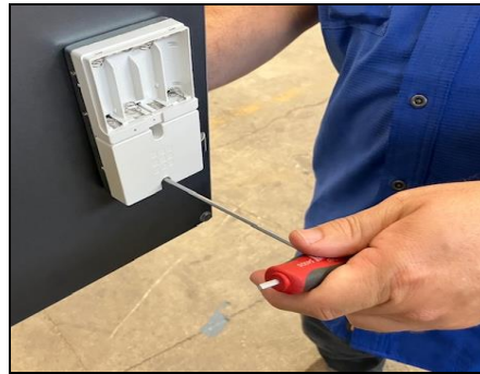
Step 9: Tighten the External Bottom Screw Verify the alignment of the ADA pull handle, then tighten the external bottom screw using a 3mm Allen wrench to secure the assembly.
