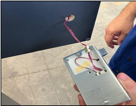
Step 8: Reconnect the Wiring to Battery While supporting the electronic lock and ADA pull handle, reconnect the wiring to the battery.
