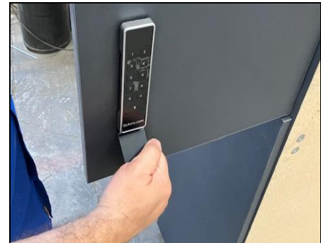
Step 13: Evaluate the ADA Pull Handle Verify that the ADA pull handle is securely installed and operates smoothly.
