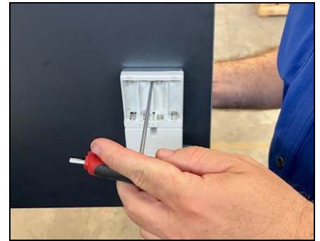
Step 10: Tighten the Internal Top Screw Confirm proper alignment is maintained. Tighten the internal top screw using a 3mm Allen wrench.
