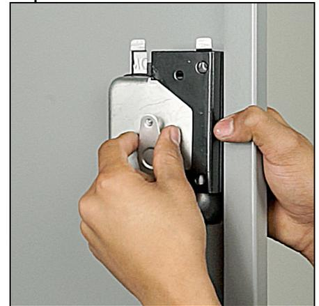
Open locker door, loosen and remove the nuts on the back of the hasp. Then remove the lock cover plate and the screws from the hasp.
